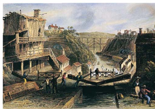
▲ A lock on the Erie Canal in Lockport, New York, shown here in an 1838 engraving, was one of 83 that helped link the Great Lakes with the Northeast.
